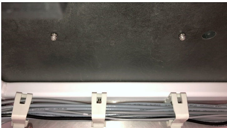
Figure 24 Condensation pump mounting screws partially installed
