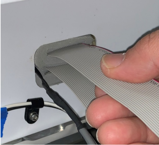
Figure 17 Pulling excess cable from enclosure formed when inserting the foam sandwich
